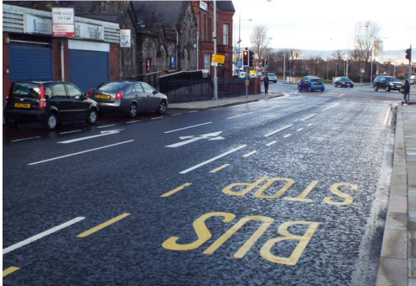
Castlereagh Street at Junction with Albertbridge Road – Widening
